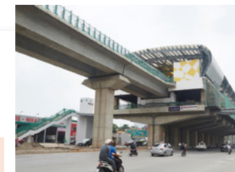
Construction of urban railway in Hanoi
