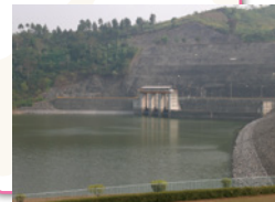
Hydraulic power generation facilities in Indonesia
