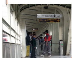
Ticket gate at BRT station in Pakistan
