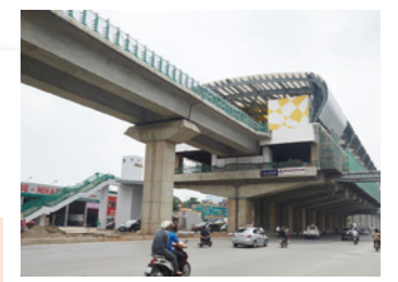
Construction of urban railway in Hanoi
