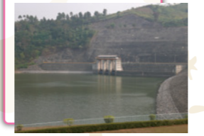
Hydraulic power generation facilities in Indonesia
